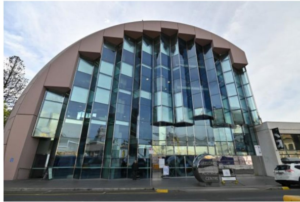
Geelong Library and Heritage Centre, (Ivan Kemp) 238448_08
